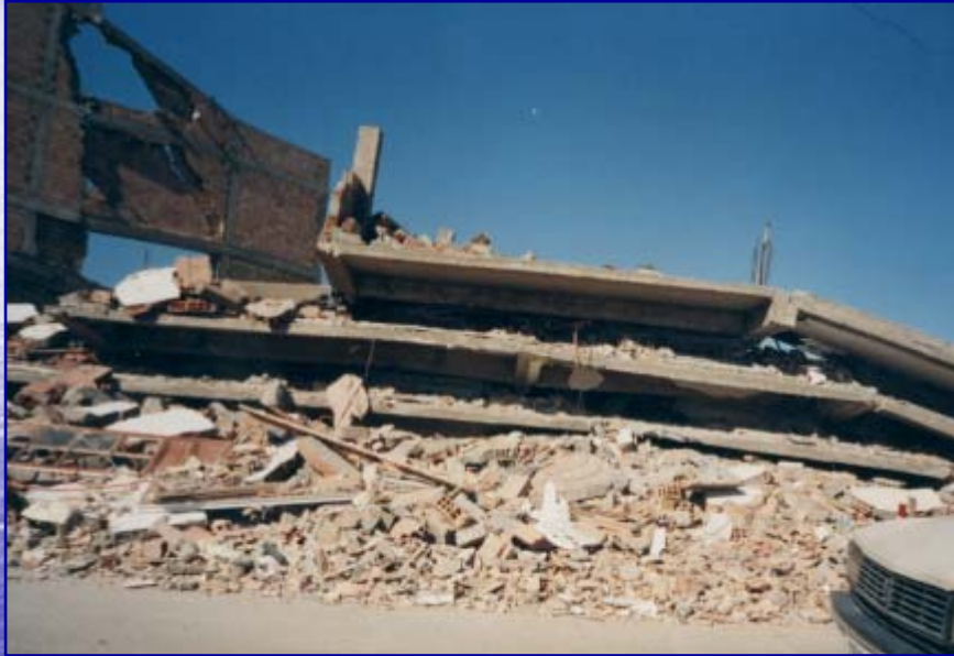
Building Damage in City of Boumerdes
