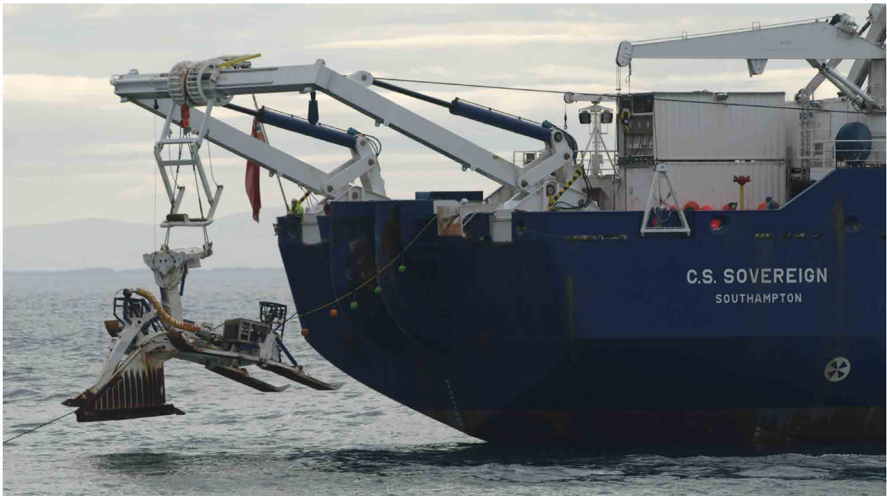
Figure 8. Cable ship with plough for cable installation. Source: Global Marine Group
