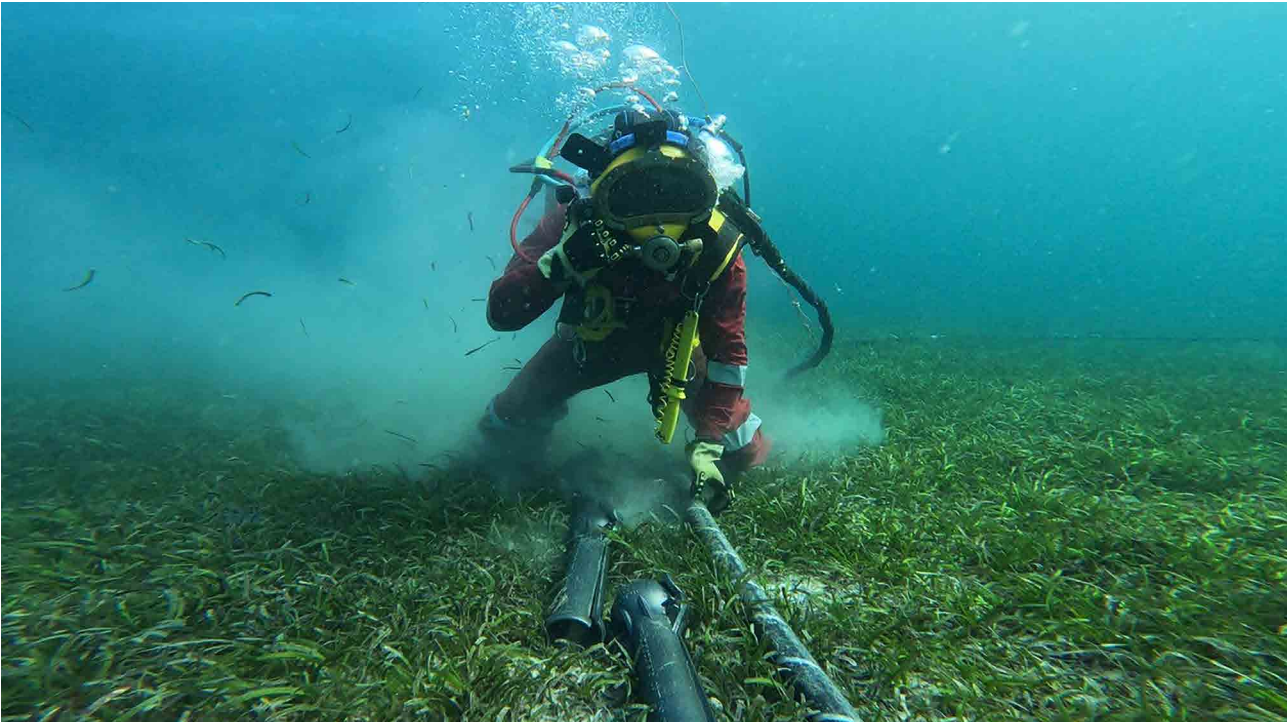
Figure 3. Scuba diver installing articulated pipe to a cable. Source: Tide & West
