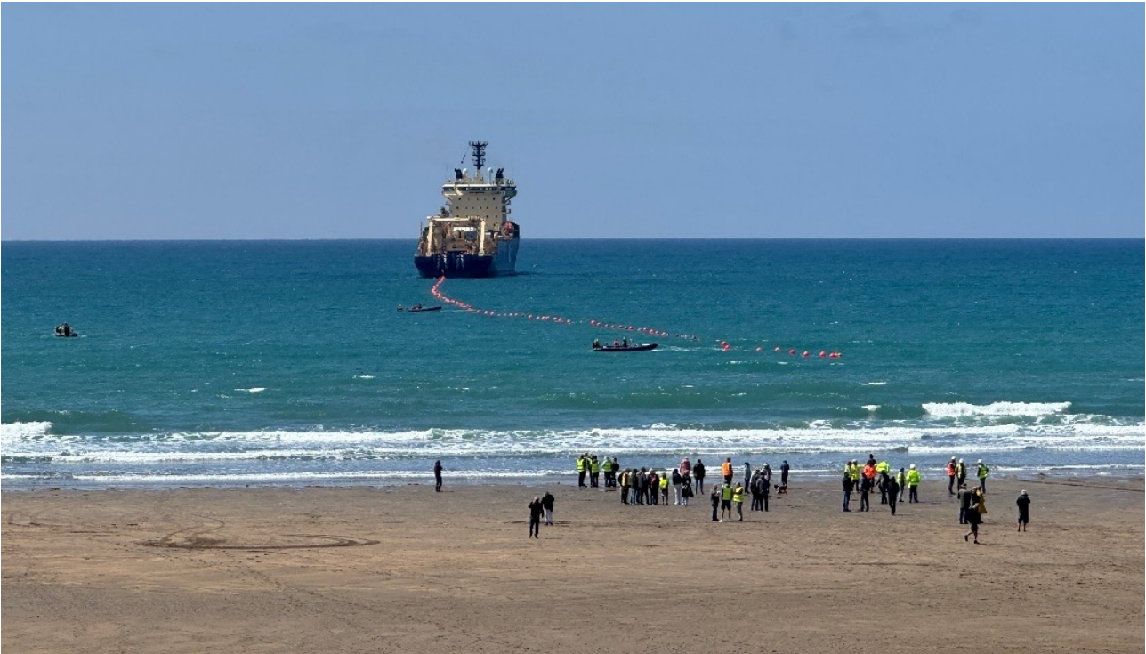
Figure 7. Direct shore end installation. Source: courtesy of ICPC
